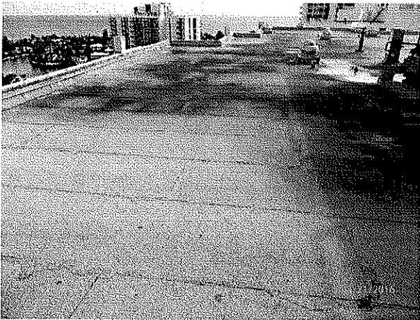
Built-Up/Rolled Asphalt Roof Covering
